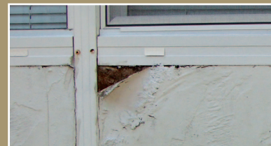
The painted aluminum used by other manufacturers scratches, sweats, and shrinks and expands with the temperature, causing gaps for heat and water leaks.
